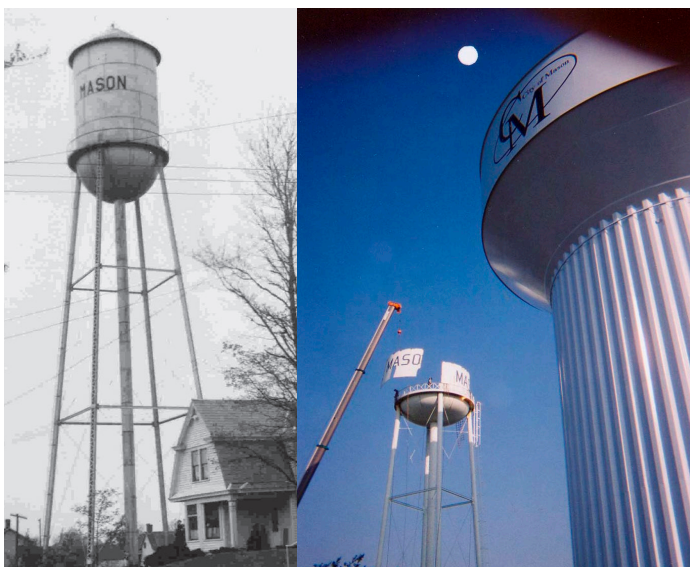
The first two towers built are no longer standing. The 1934 West Church St. tower (left) was dismantled in 2004. The 1956 Kings Mills tower (right) was also dismantled the same year, following the completion of a new tower, 20 times its predecessor's size.
